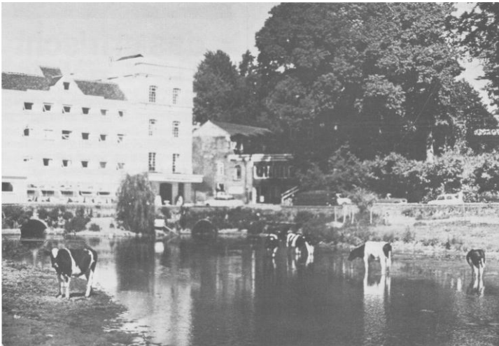
Mill-Hotel in Sudbury
